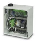
Measurement system for load characteristics and bending moments in rotor blades of wind turbine generators. Proactive rotor blade monitoring, early detection of damage, and optimized load control. Reliable in harsh ambient conditions and suitable for remote service.
